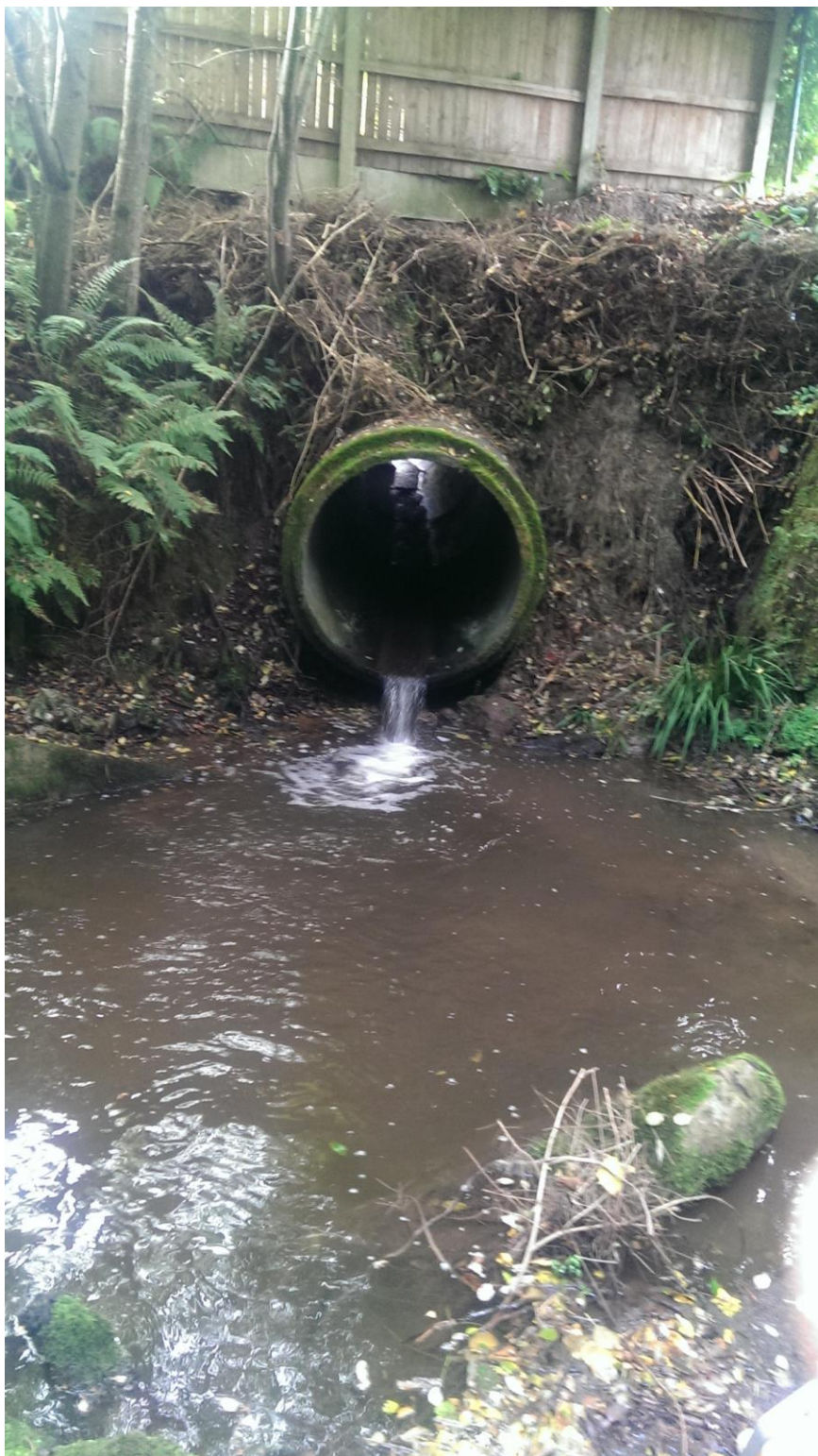
Photo 2. Plunge pool and pipe which forms a further barrier to fish movement at the upstream end of Site 1.
